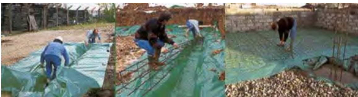
photo 16: pose du Termifilm®. (91)
